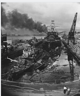
Pennsylvania , behind the wreckage of Downes and Cassin
