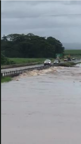
The North Johnstone Bridge on the Bruce Highway
