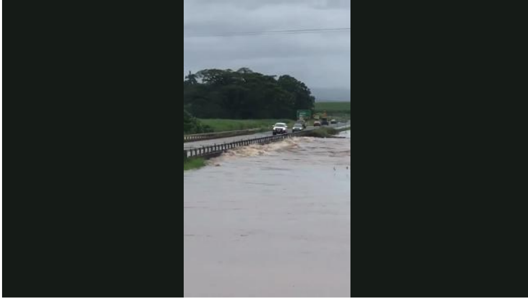
The North Johnstone Bridge on the Bruce Highway
