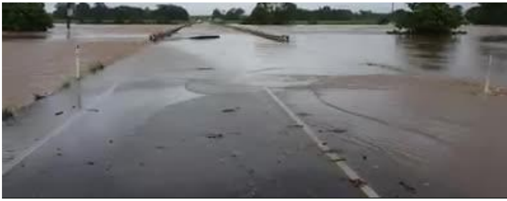
North Johnstone bridge closed
