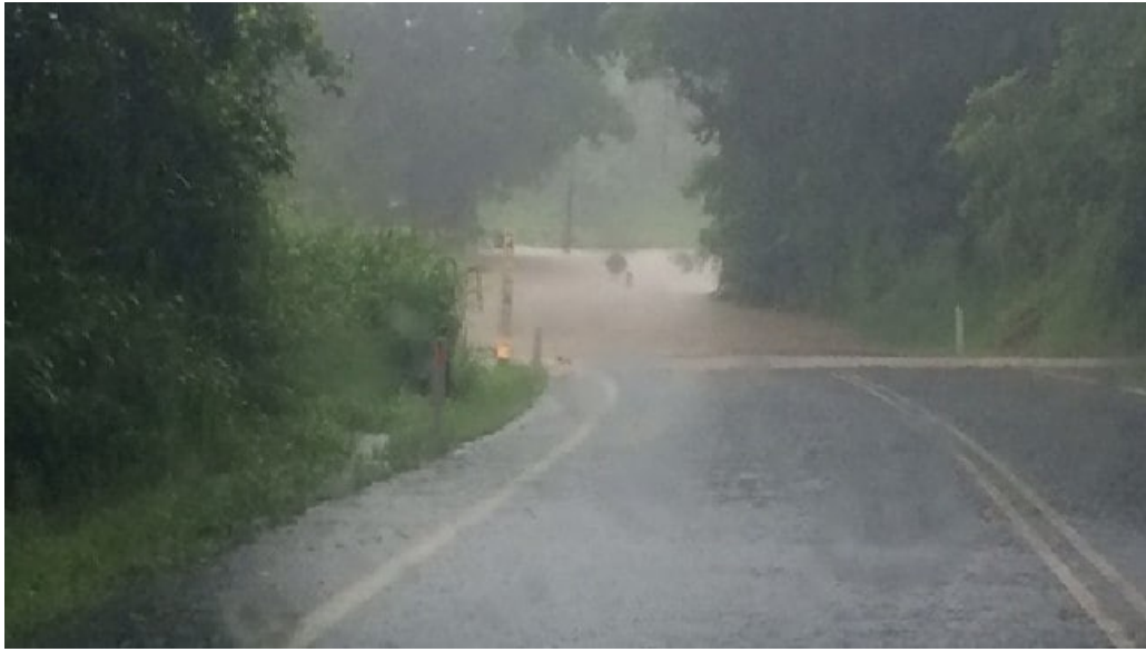
📷 Gillies Highway (including the Gillies Range) is presently closed due to flooding. The highway is closed from Vico Road at Gordonvale, through to Boar Pocket Road on the Yungaburra side of the range.
